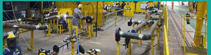
SUBSEA SPOOLS AND RISERS WELDING PROCESS
